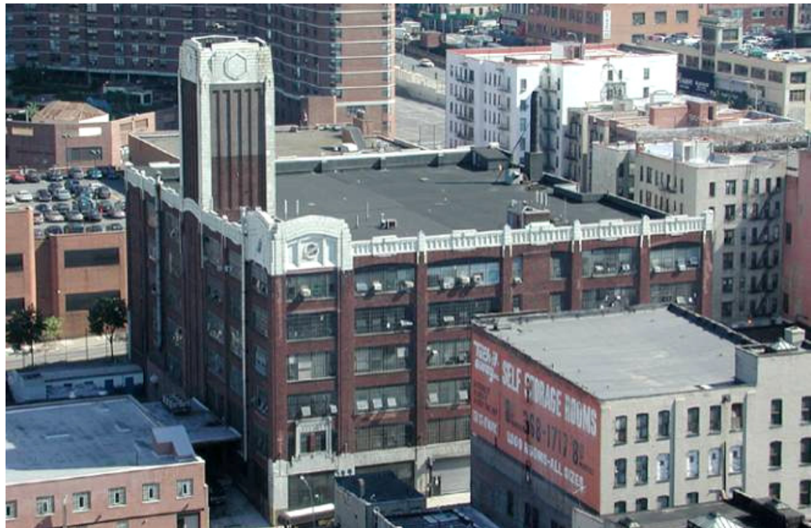
The Studebaker Building 615 W. 131st Street
