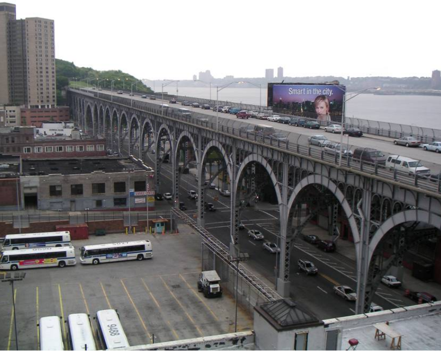
Looking South 12 th Avenue / Riverside Drive Viaduct
